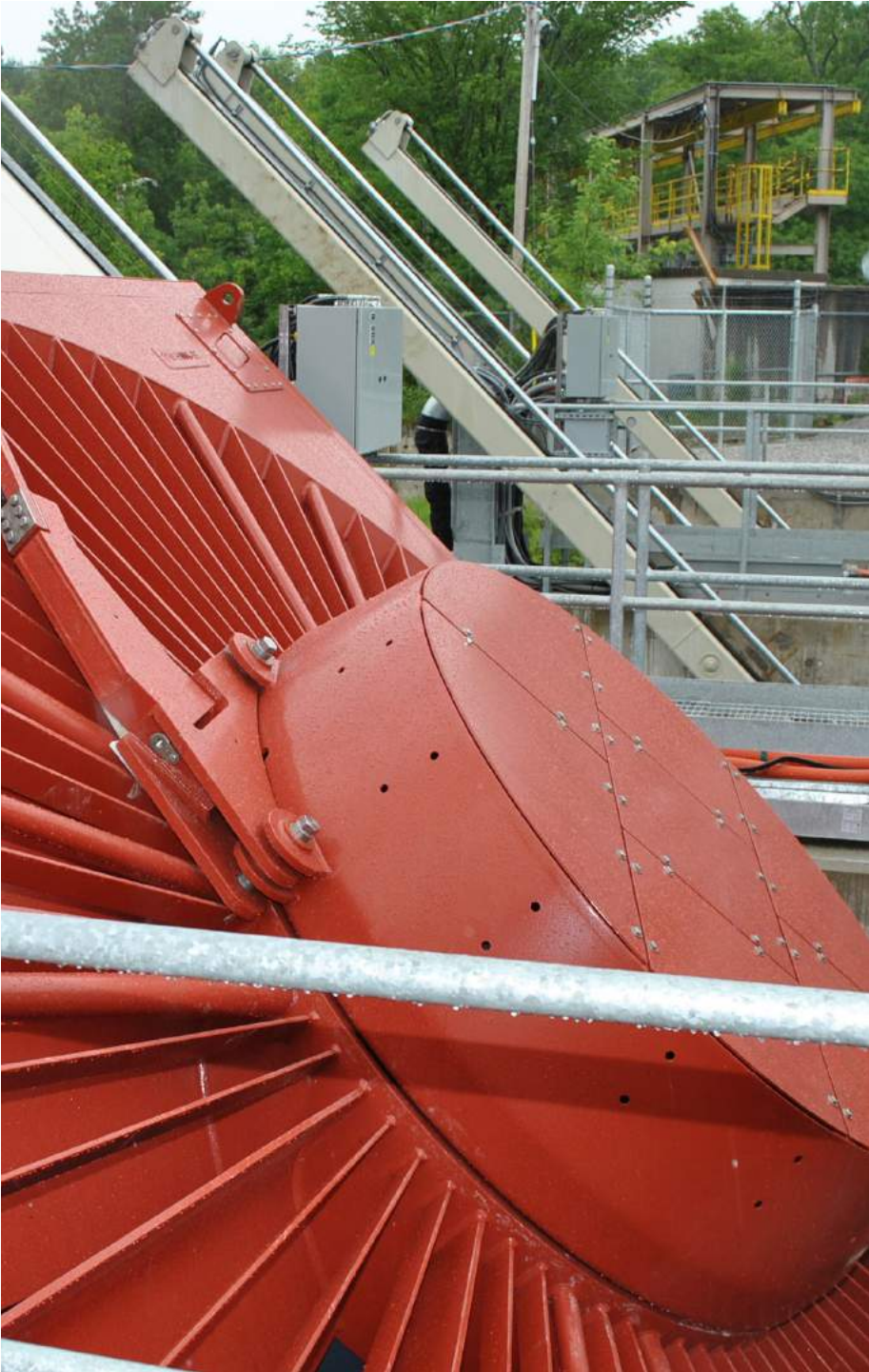
Figure 27: Wasdell Falls Generating Station (1.65 MW) - Wasdell Falls Limited Partnership (WFLP) - Very Low Head (VLH) Turbine
