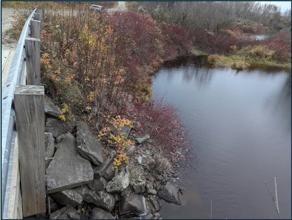
16. B-030 2024-10-23 Southwest Embankment
