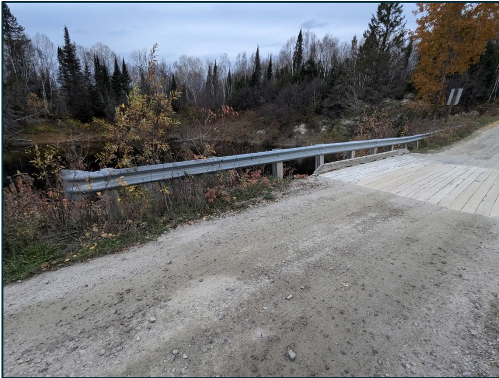
5. B-030 2024-10-23 West Barrier Over Structure
