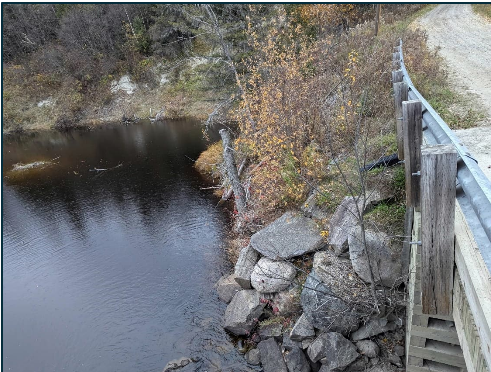
14. B-030 2024-10-23 Northwest Embankment
