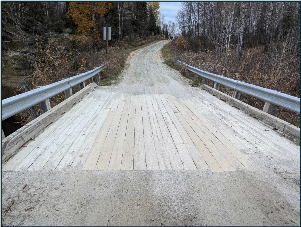
7. B-030 2024-10-23 Deck Looking North
