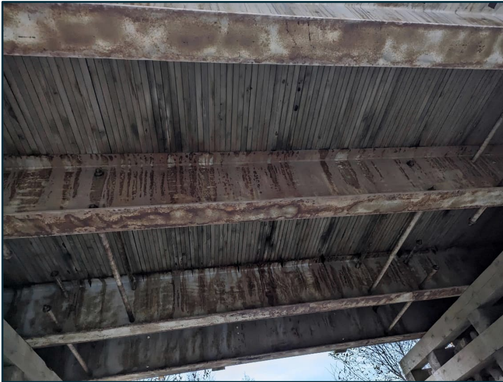
9. B-030 2024-10-23 Girders and Soffit Typical
