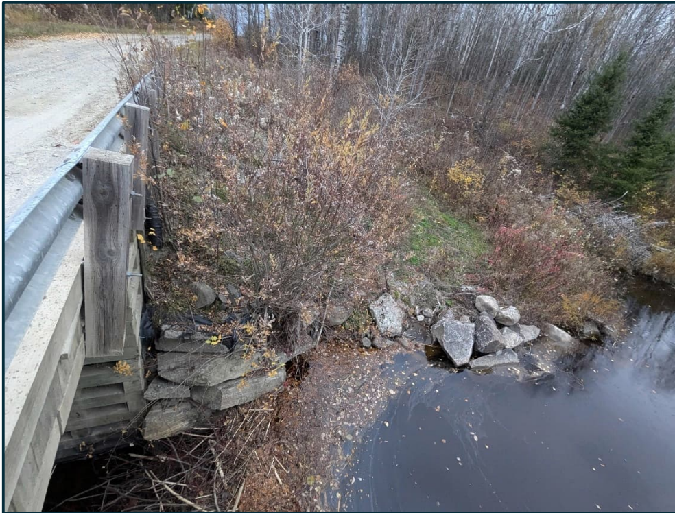
13. B-030 2024-10-23 Northeast Embankment
