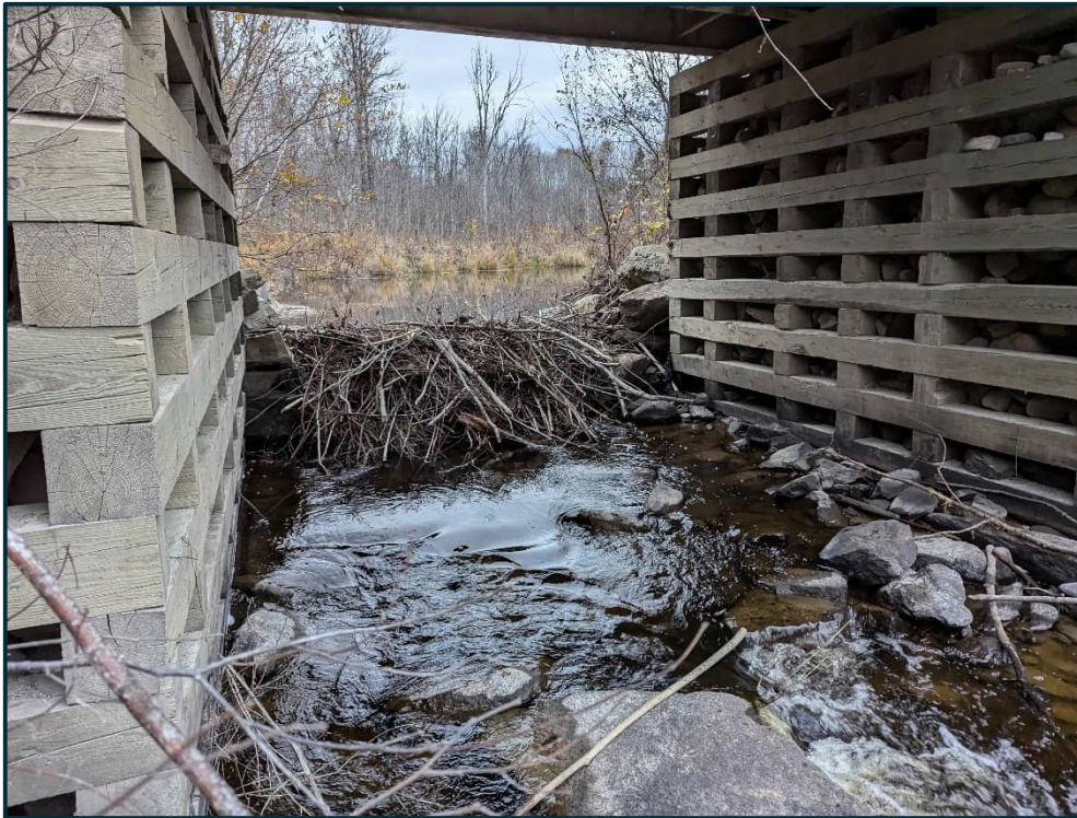
19. B-030 2024-10-23 Bever Dam Below Structure
