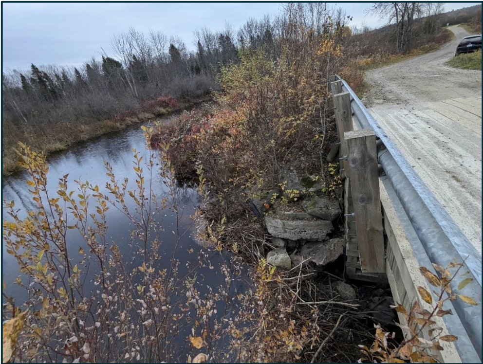
15. B-030 2024-10-23 Southeast Embankment
