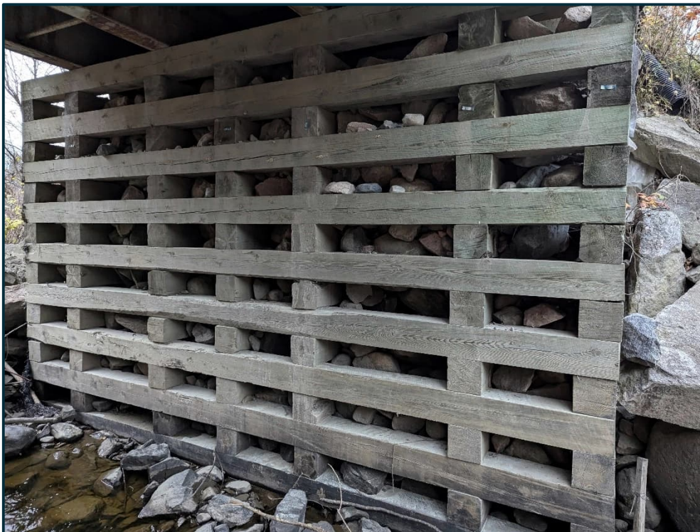
12. B-030 2024-10-23 South Abutment
