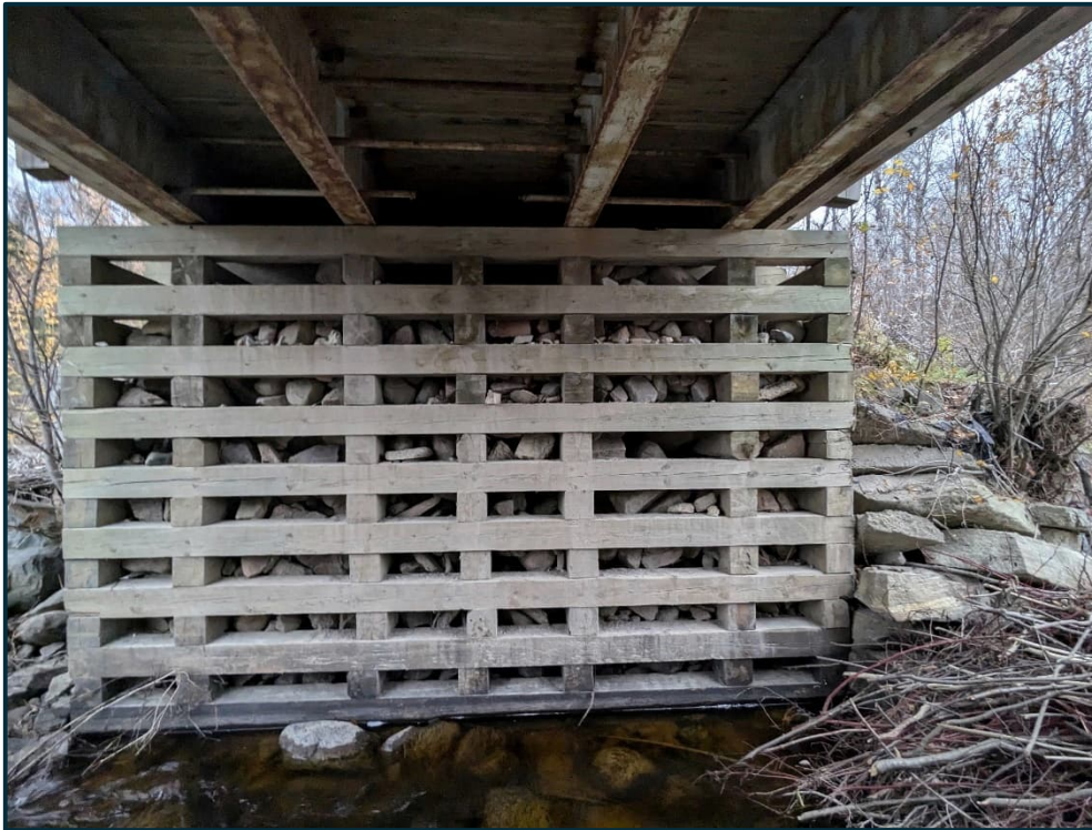
11. B-030 2024-10-23 North Abutment
