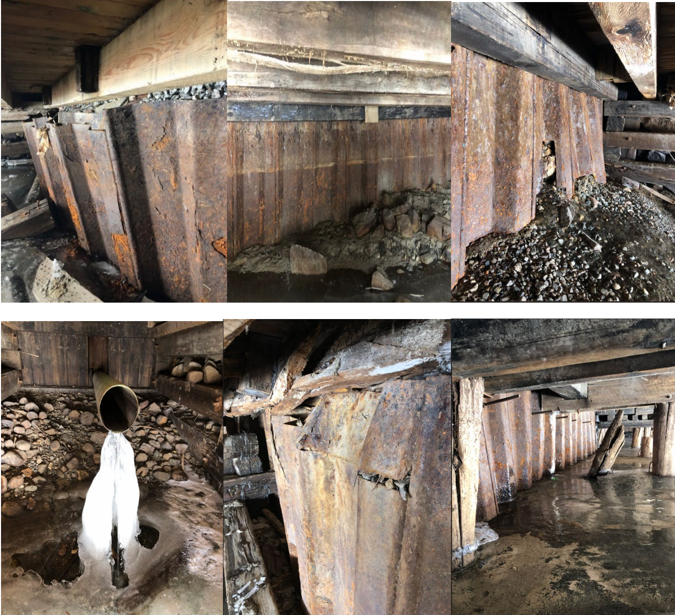
Typical sheet pile between wharf and road
