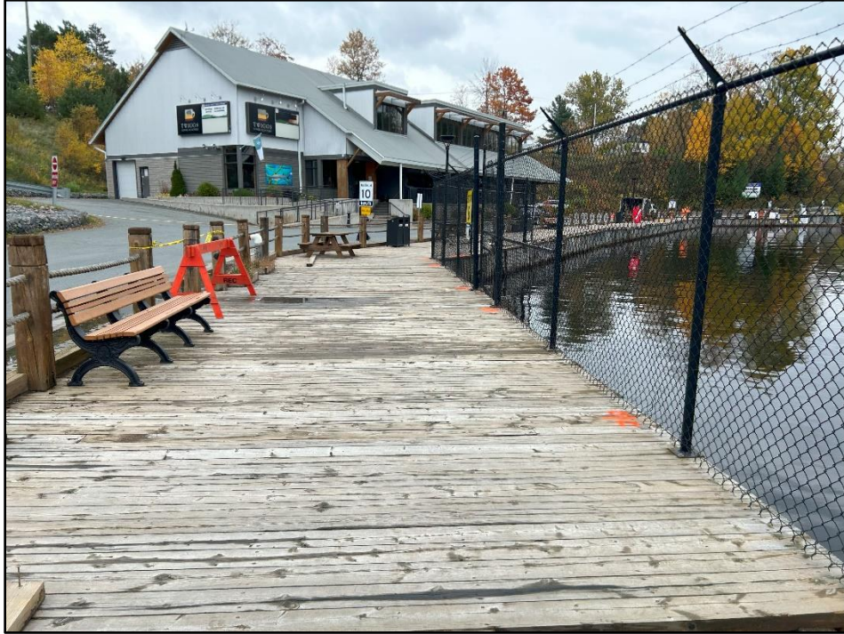
Photo 11: Wood decking near Station 240.
