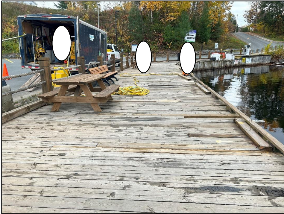
Photo 15: Wood decking near Station 445.
