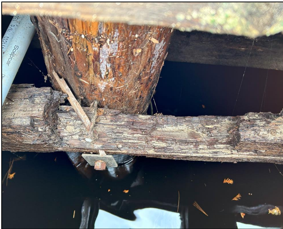
Photo 41: General wood bent pier and header attachment.
