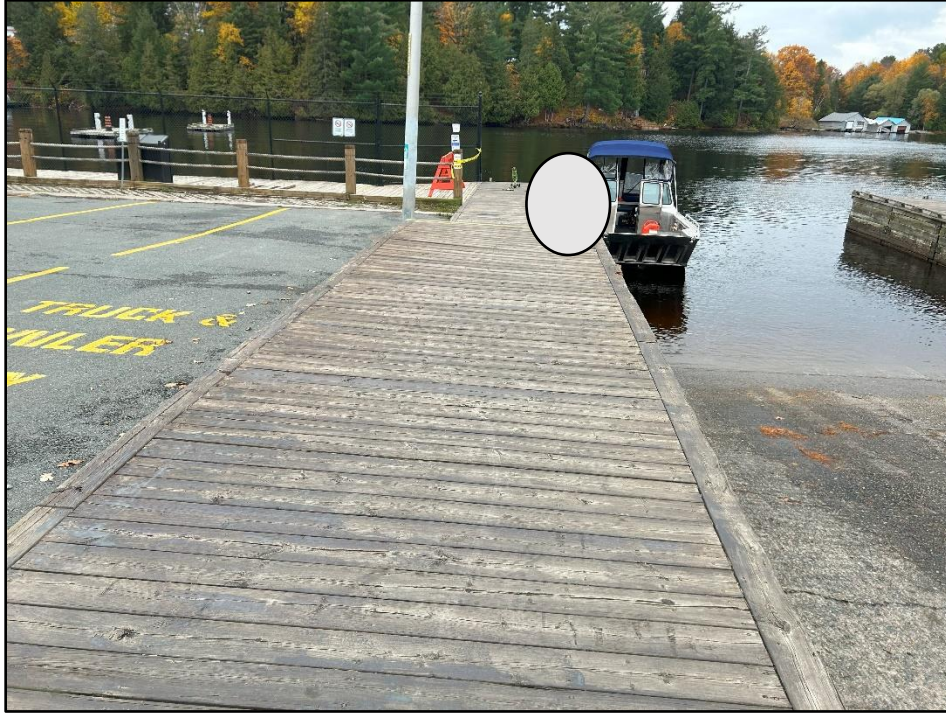
Photo 5: West end decking near boat launch ramp.
