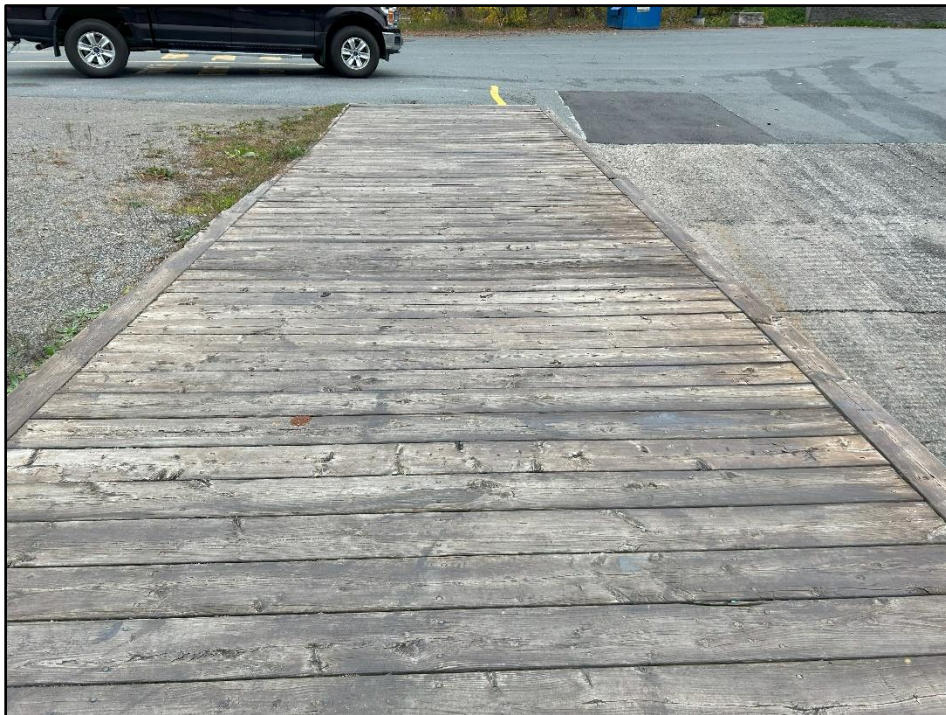
Photo 4: West end decking, near boat launch ramp.
