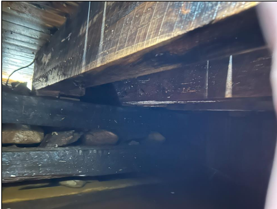
Photo 30: General stringer condition near Station 247.
