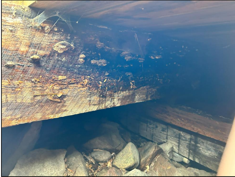
Photo 31: General stringer condition near Station 255.
