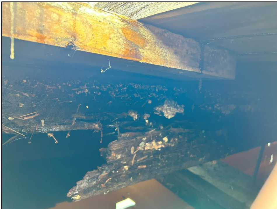
Photo 34: General stringer condition near Station 350.
