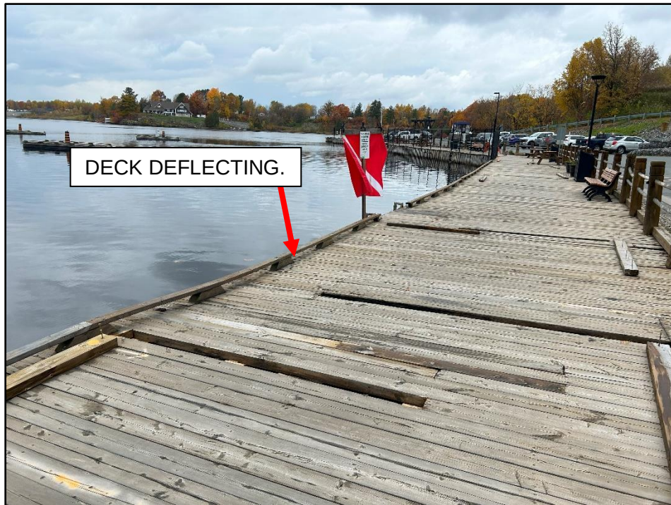
Photo 14: Wood decking near Station 310.
