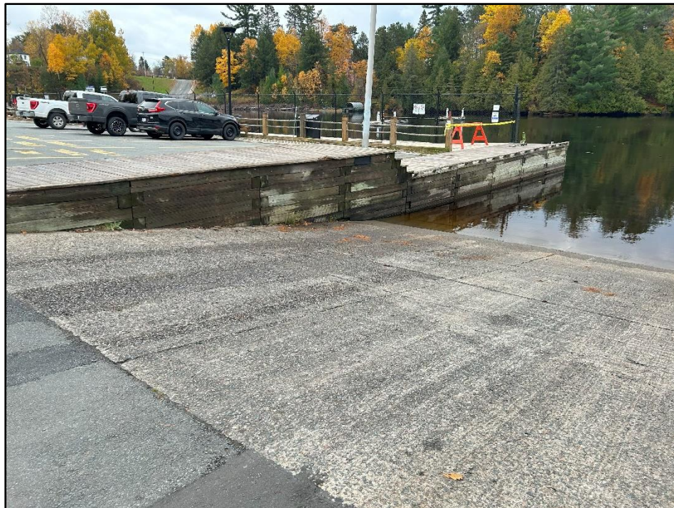
Photo 18: General view of boat launch concrete ramp.
