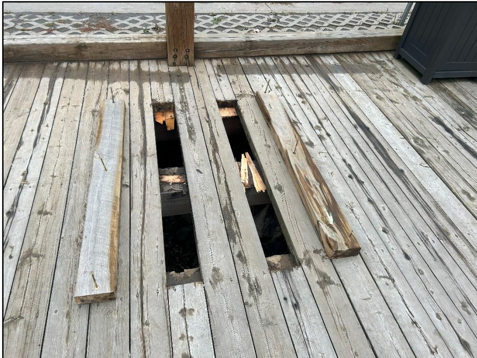
Photo 8: Wood decking near Station 0.
