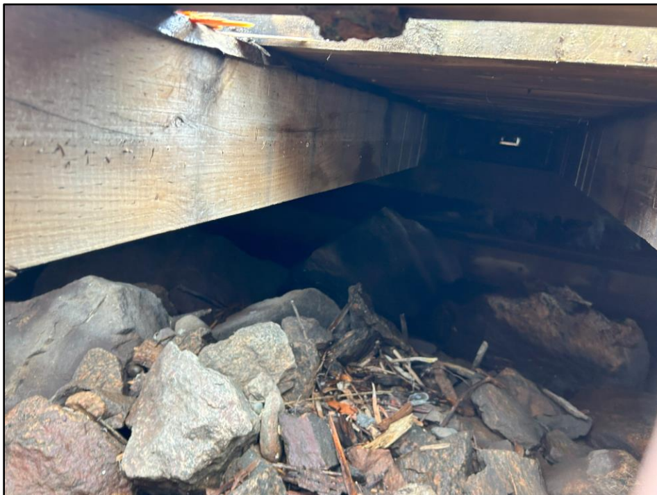
Photo 26: General stringer condition near west end.
