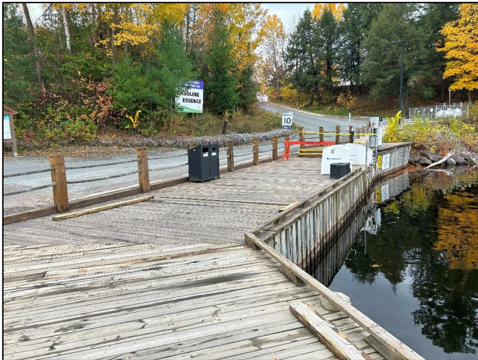
Photo 16: Wood decking near Station 515.
