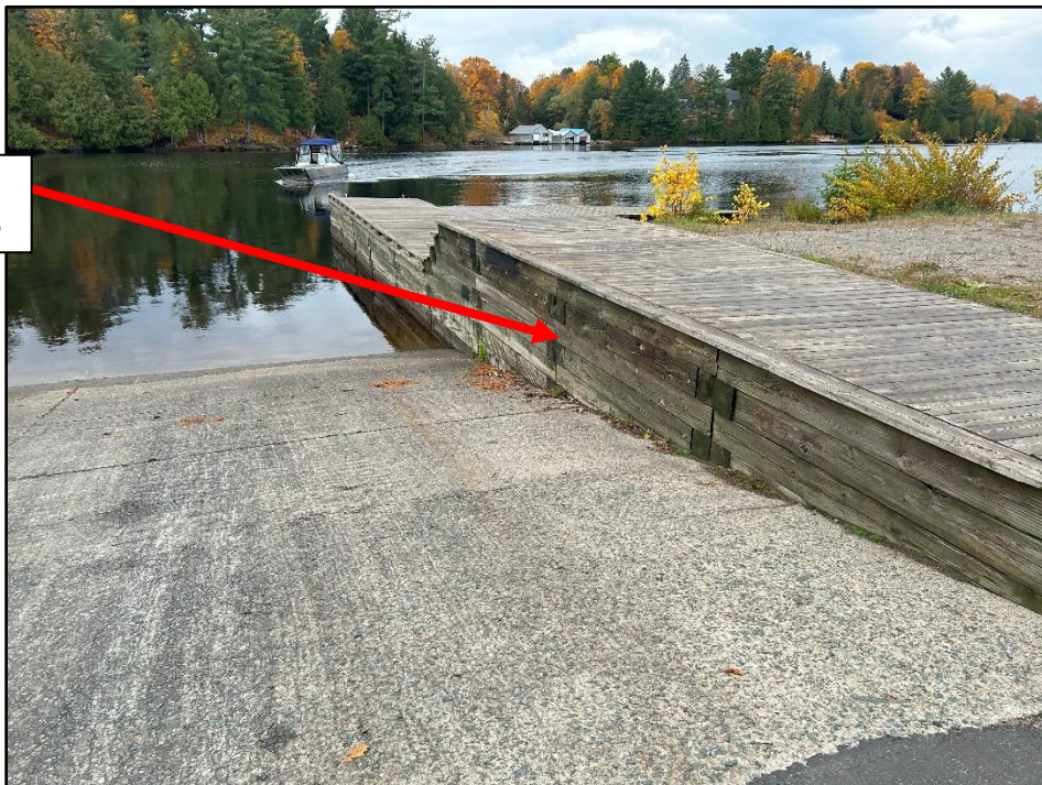
Photo 20: General view of boat launch side wall cribs.
