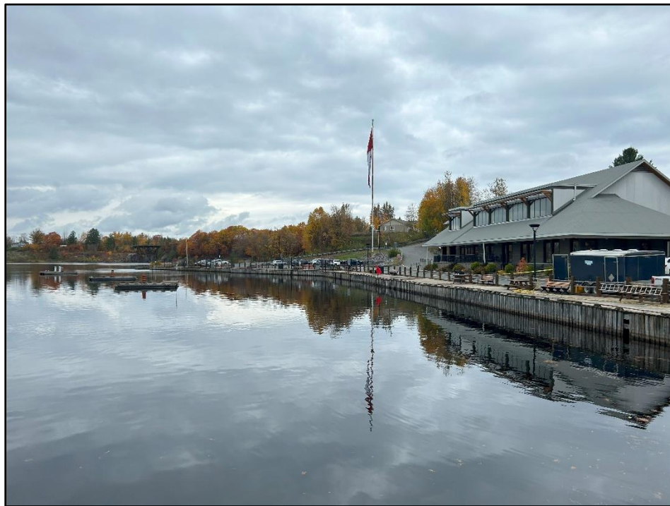
Photo 2: East exterior elevation, looking north-west.
