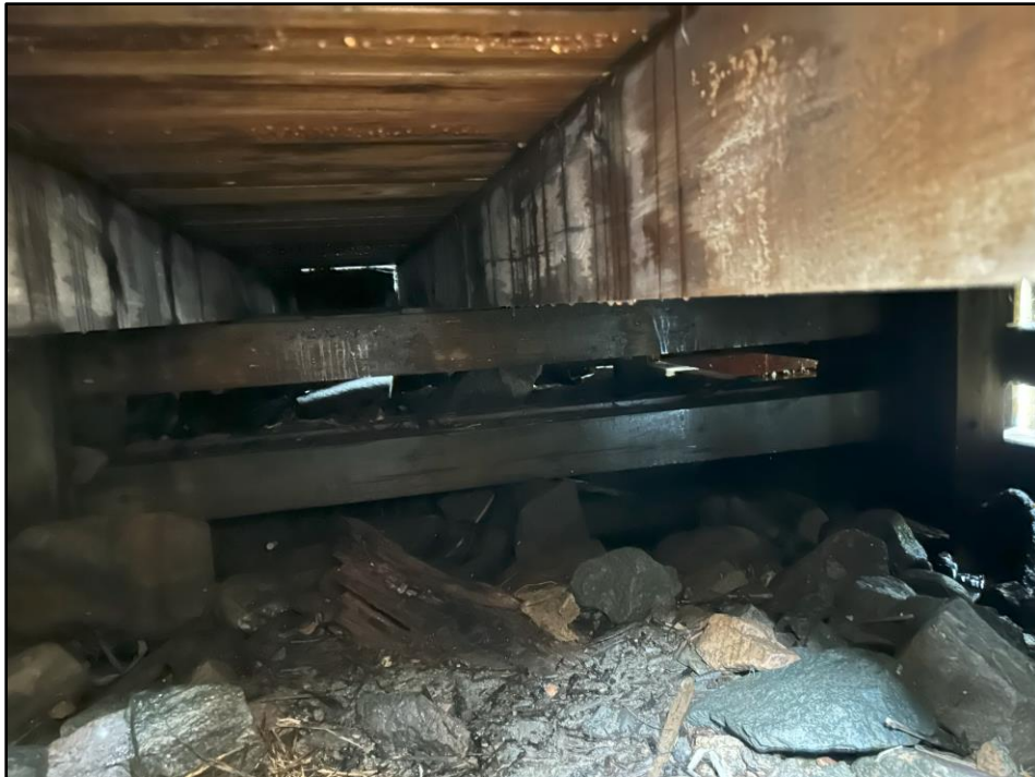
Photo 28: General stringer and crib condition near Station 134.
