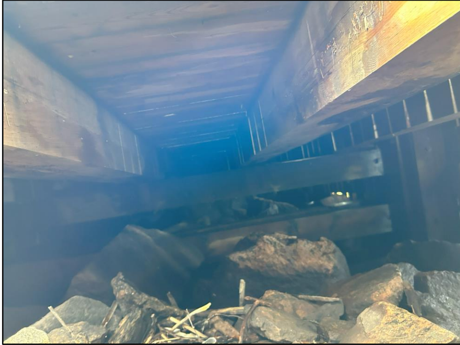
Photo 27: General stringer condition near west end.
