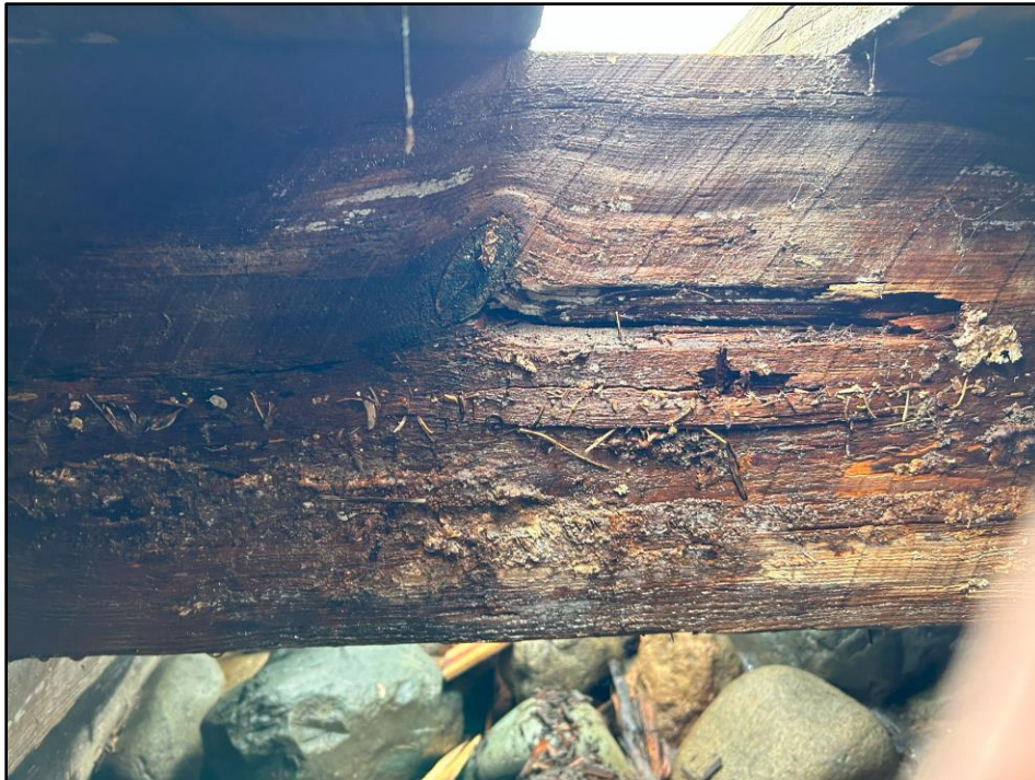
Photo 32: General stringer condition near Station 255.
