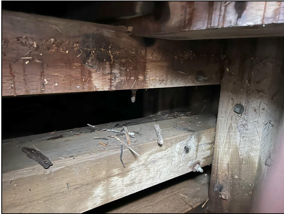
Photo 39: General cribbing condition near Station 134.
