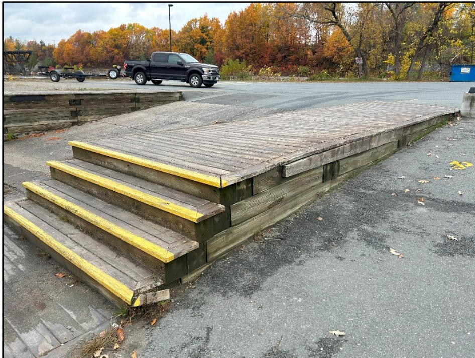
Photo 6: West end decking near boat launch ramp.
