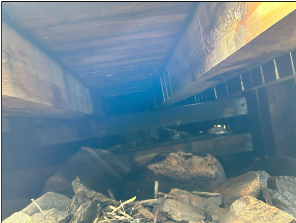
Photo 38: General cribbing condition near west end.
