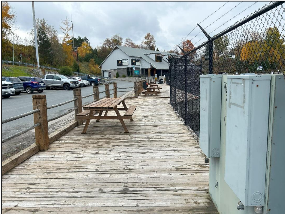
Photo 10: Wood decking near Station 134.
