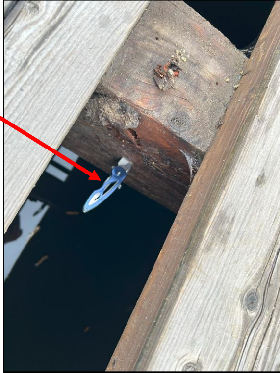
Photo 37: General stringer condition near Station 515.
