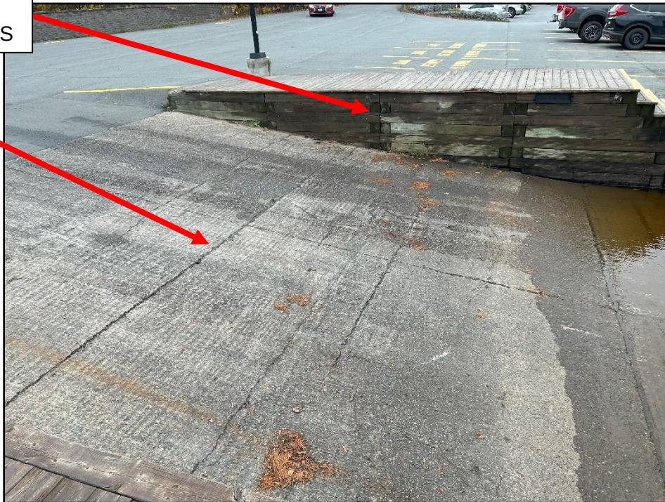
Photo 19: General view of boat launch concrete ramp.
