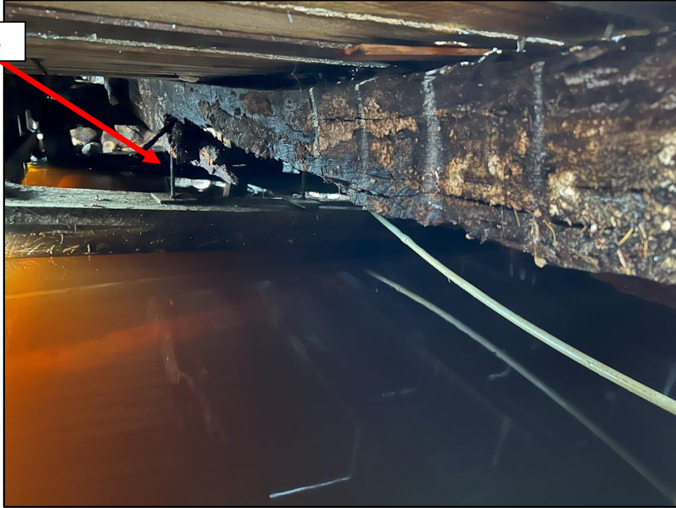
Photo 33: General stringer condition near Station 350.
