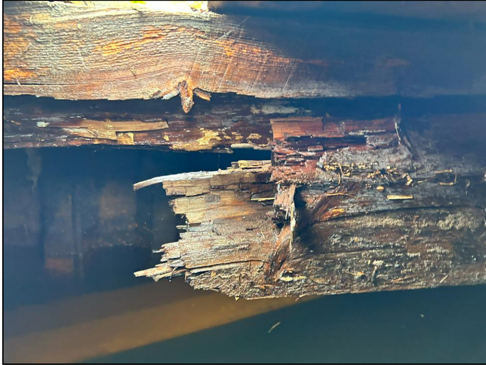
Photo 35: General stringer condition near Station 350.
