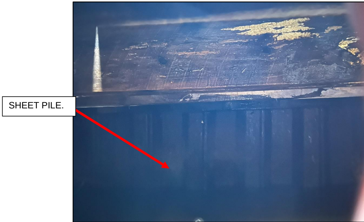
Photo 42: General sheet pile.
