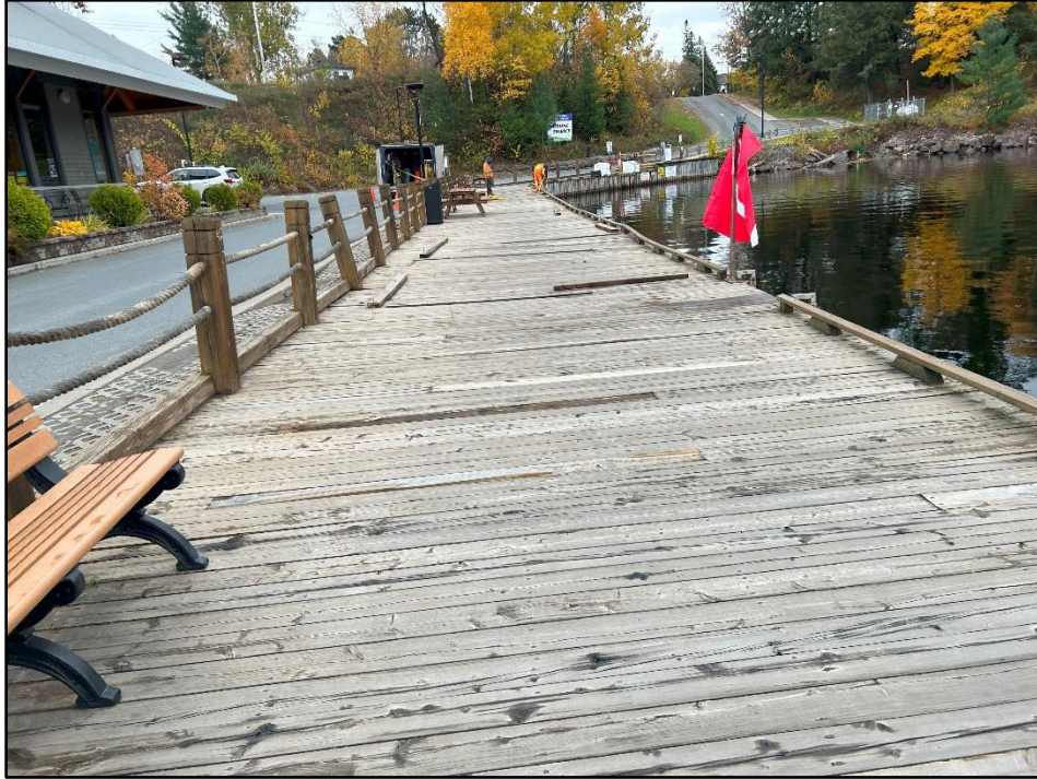
Photo 13: Wood decking near Station 300.
