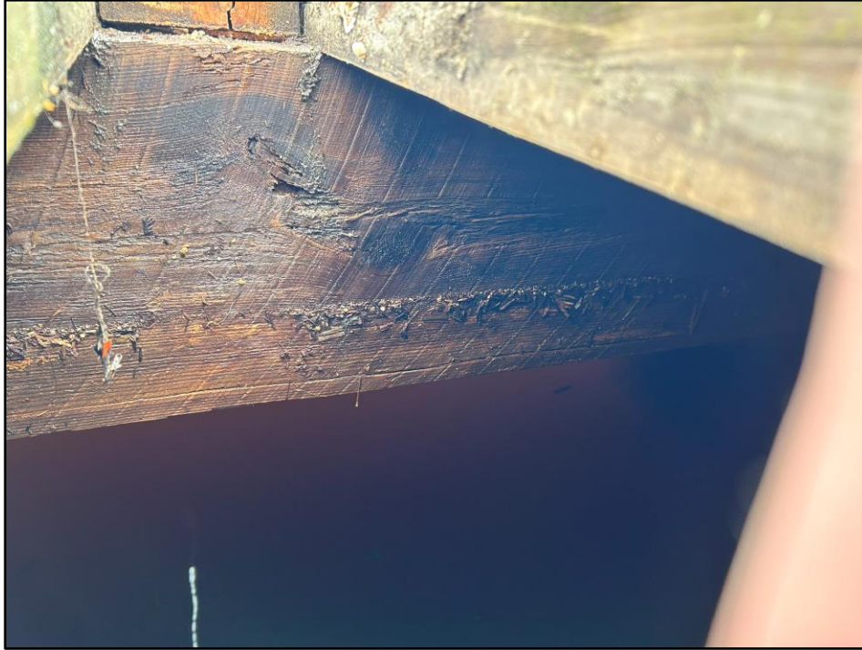
Photo 29: General stringer condition near Station 247.
