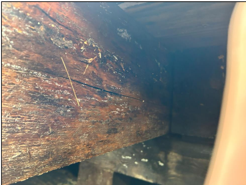
Photo 36: General stringer condition near Station 515.
