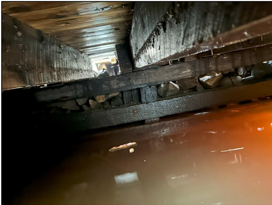
Photo 40: General cribbing condition near Station 150.
