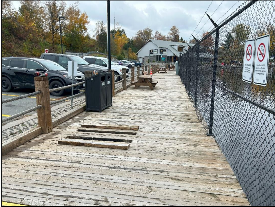
Photo 7: Wood decking near Station 0.
